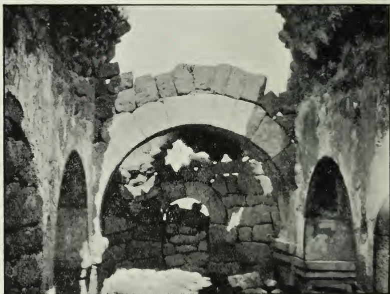
FIG. 106.—No. 16, interior of apse.
